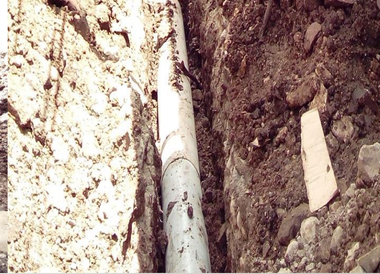
construction of inspection chambers
