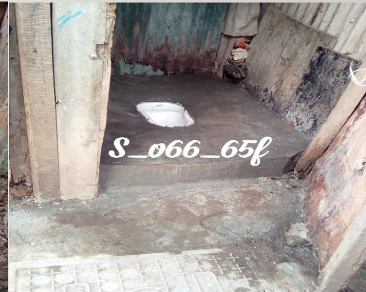
Upgrading of toilet
