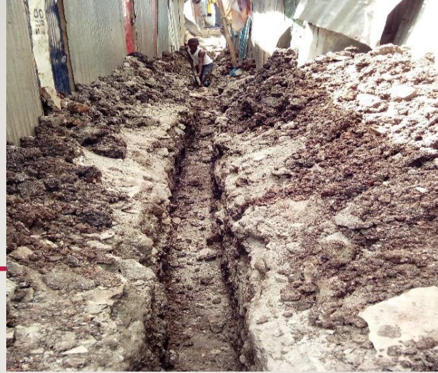
sewer route excavation
