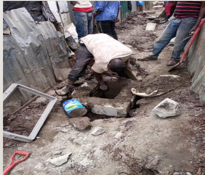
sewer pipe lying
